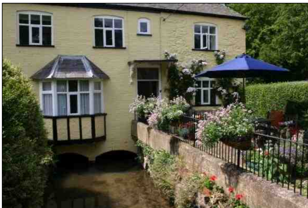
Figure 12: The Ginge Brook at Lower Mill during low flow conditions.
