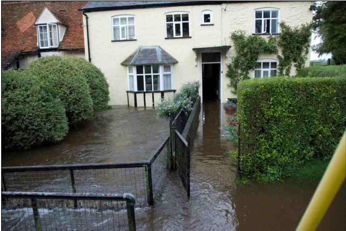
Figure 8: Flooding of the Ginge Brook in Sutton Courtenay, July 2007.
